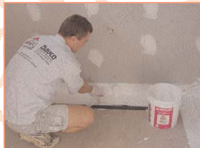
Newington Village, Homebush, NSW - Waterproofing wet areas using Davco Dampflex Waterproofing Contractor: R+R Fibreglass Flashing (Nthn Div) Builder: Mirvac Group
